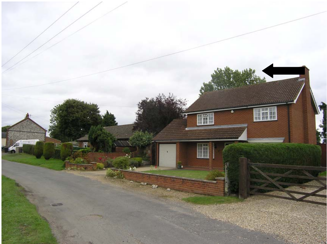
T1, Viewed from the junction Of Mere Road.
